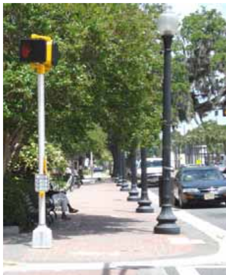
Example of a sidewalk separating pedestrians from vehicles with texture color and light poles.
